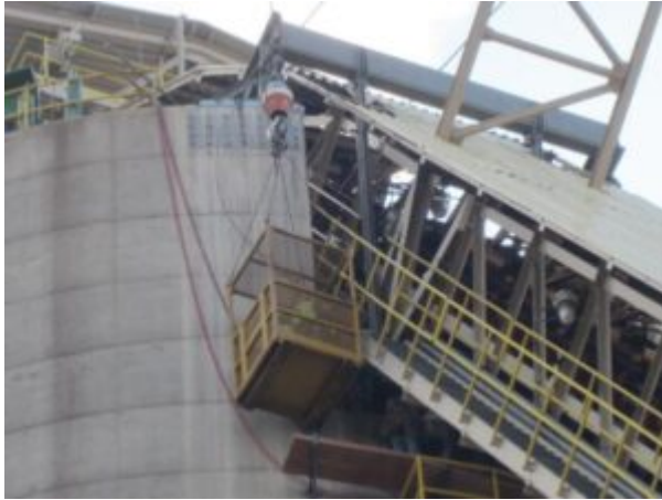
Figure 3: With the new upper support system complete, the HAC is ready to resume productive operation.
