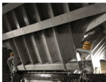
Figure 1: Hollow structural sections used to resist moment and torsion created by new feeder loads.
