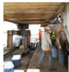
Figure 2: Temporary steel support
